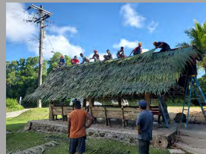
Both koyeng roofs were replaced by many of the church members working together to weave the thatch and tie the bamboo pieces to the roof. Truly and Jack also replaced the tin roofs on the apartment and Sunday School room.
