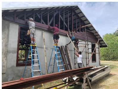
Installing local mahogany siding
