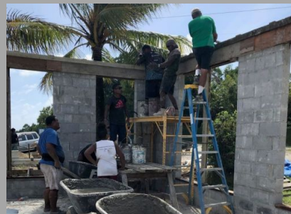
Pouring the Beam in early January
