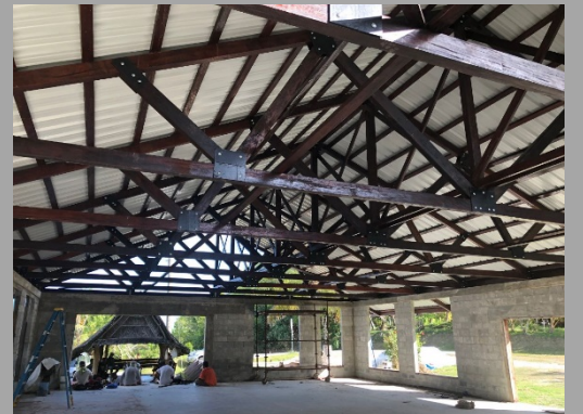
Interior view of exposed beams
