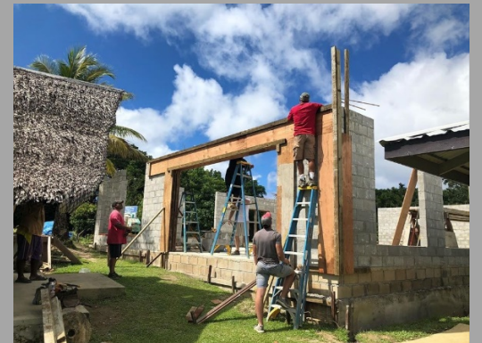
Making forms over garage-door opening
