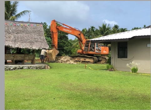
Ground Breaking for new building
