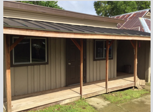
New porch on the apartment
