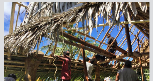
Men putting on roof
