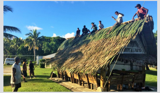
Men on top of nearly finished roof
