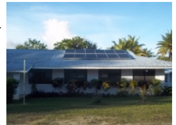
Church Solar Panels
