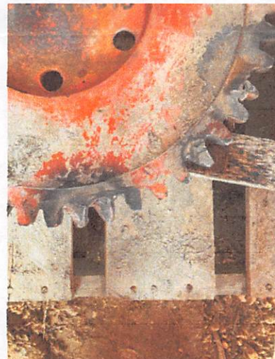
Repaired Gear teeth of cement mixer
