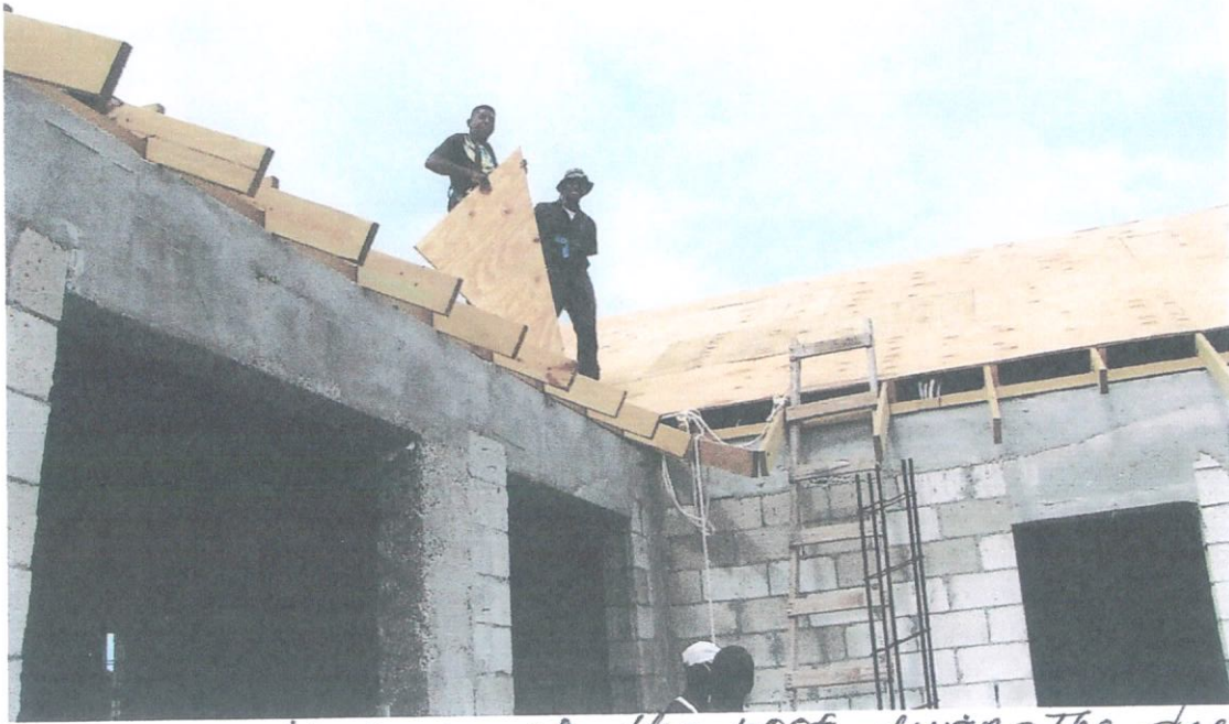
Helping on the roof during the day
