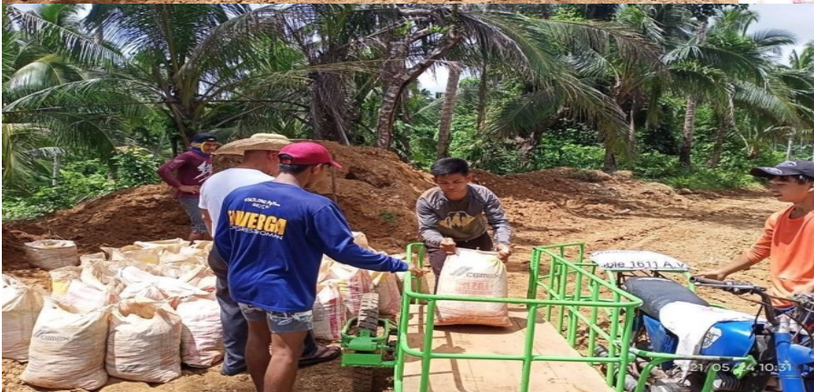
Pastor Elmar, Pastor Jerime and the construction crew are working to raise the level of the property where the new church building will be built. With the typhoon season and frequent flooding, it will help prevent many problems.
