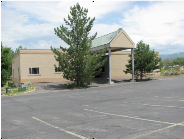
South side of building; property line extends 19' from pillars. Lined parking spaces belong to IHC hospital.
