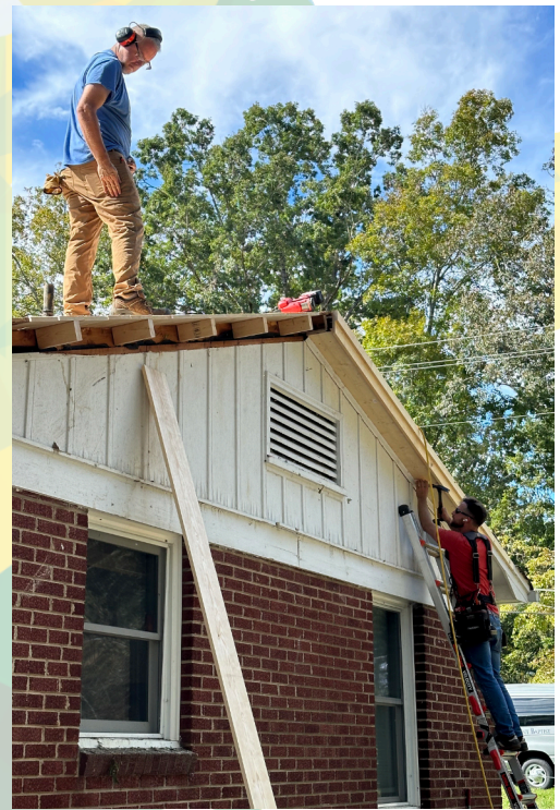
Others helping repair the damage on our home!
