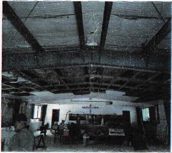
Stripped ceiling on both pew and pulpit sections. The plan is to raise it up to top of I-beam.
