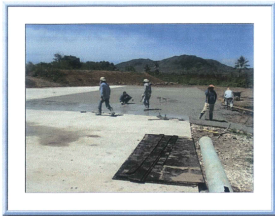
Pouring the cement for the parking area
