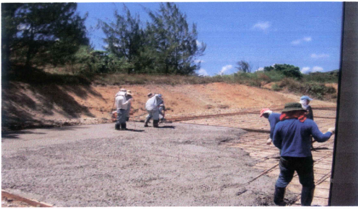
First pouring of the parking area.
