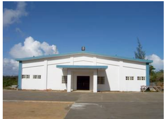
Main entrance to the building, partially paved parking area.
