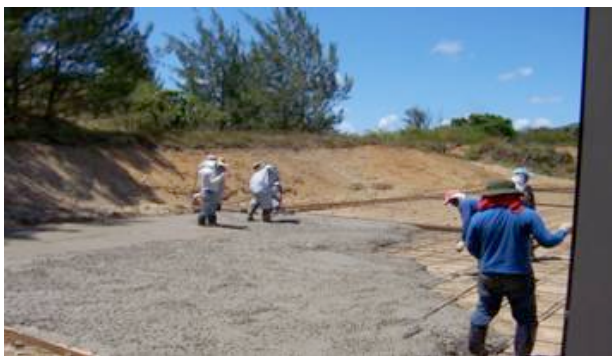
First pouring of the parking area.
