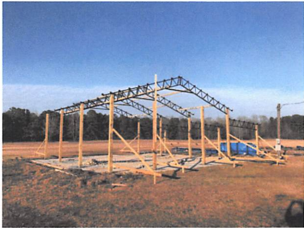
Pole Shed coming along ...
