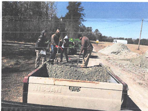
Young men refurbishing our 1 mile road
