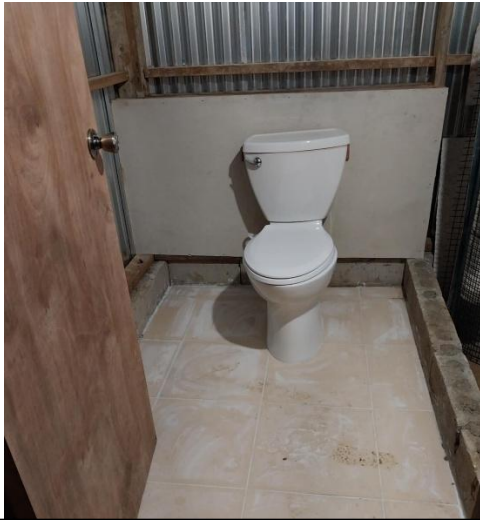
Our newly restroom building
