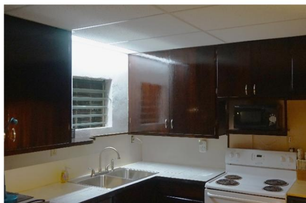
Putting the finishing touches on the renovated kitchen, dining, and living areas!
