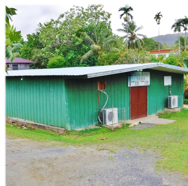
New roof on the Calvary Baptist Church
