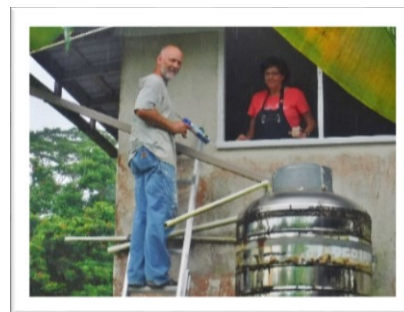
Station repairs, rain or shine!
